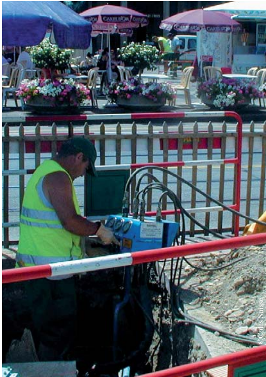
Replacement of pipes by bursting.
